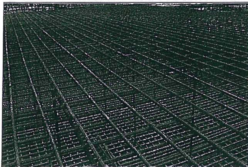
Figure 5-5 Binding of Foundation Rebars
